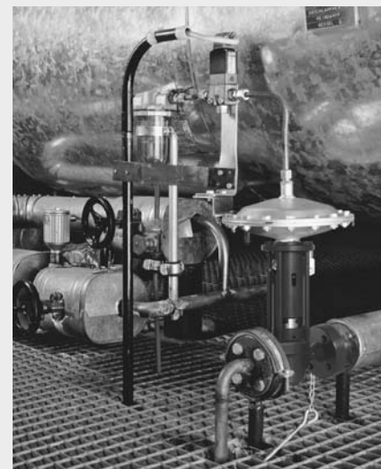
Automatic intermittent blowdown with the GESTRA MPA
